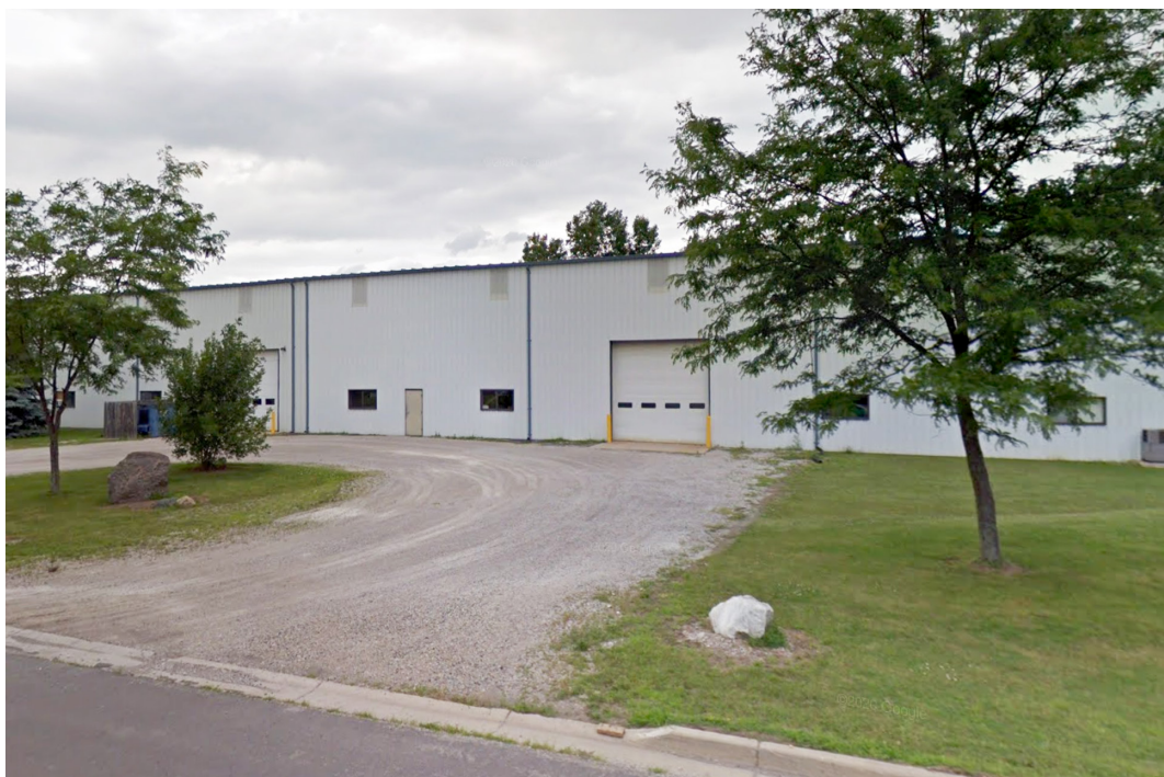
A property in the industrial park.
