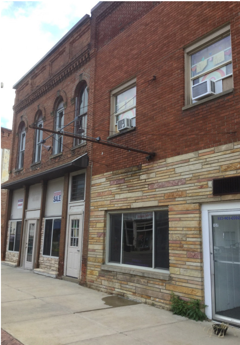
Downtown facades have a mix of building materials.
